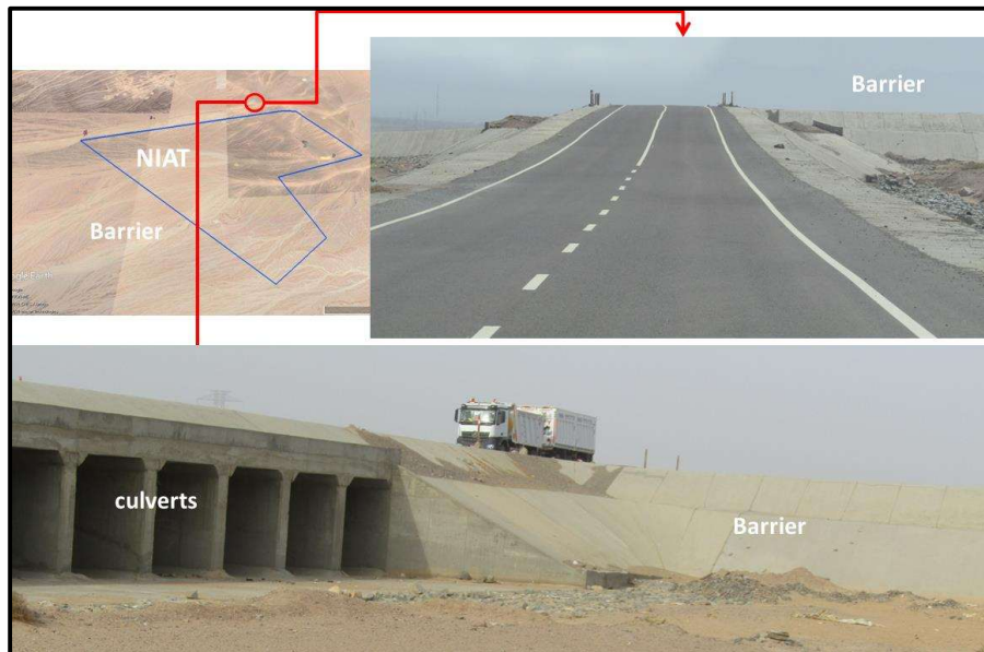
Figure 88: Field photographs of Water Barrier at 8km Mark and Associated Culverts
