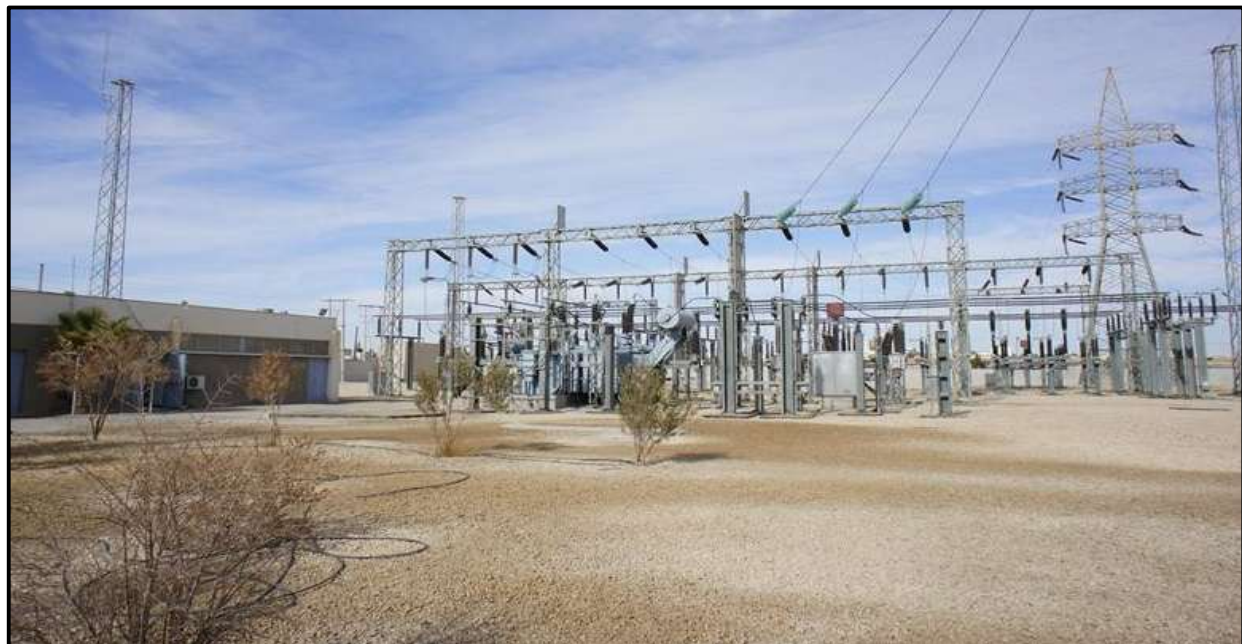
Figure 9: Typical 33/220kV Substation
